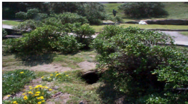
Exposed Drain prior to enviromedia installation
