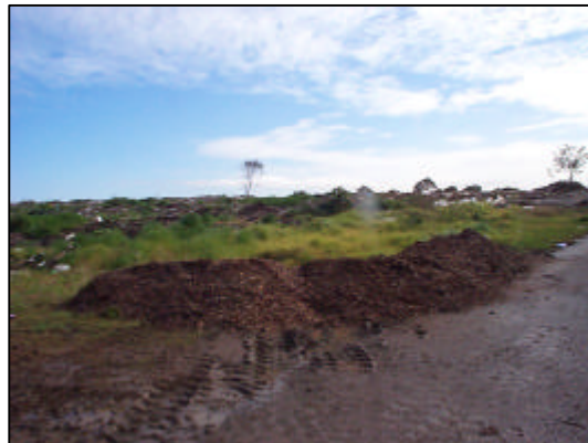
Freshly chipped RO formed into a berm
