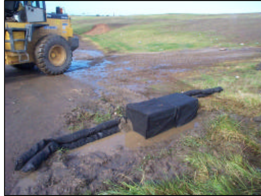
Installation of devices containing RO
